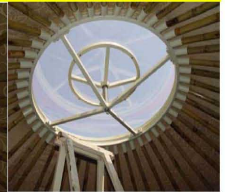
11. Screw the skylight into the hole of the center ring and make them together and strong, you can also leave a little space between each other to keep ventilated.
