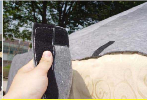
7. Add the several cotton felts as the second inner cover, and use velcro connect with each other. It can keep heat preservation function.
