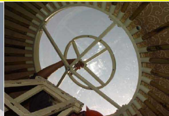
11. Screw the skylight into the hole of the center ring and make them together and strong, you can also leave a little space between each other to keep ventilated.
