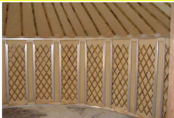
12. See the door and inside of the yurt, the lattice wall made from so many strong bamboo and the rafters is made from 3cm diameter bamboo.
