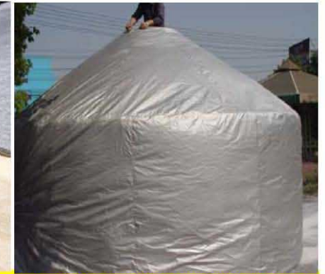
8. Add the cloth plated with silver as the third cover, and it can prevent ultraviolet radiation.
