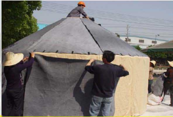
7. Add the several cotton felts as the second inner cover, and use velcro connect with each other. It can keep heat preservation function.
